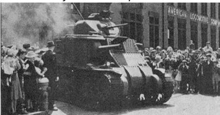
In early 1940, the first M3 medium tank to be produced by a private industrial company emerges from the American Locomotive Co., Schenectady, NY. The M3 is armed with a 75mm gun and powered by a Wright airplane engine.
